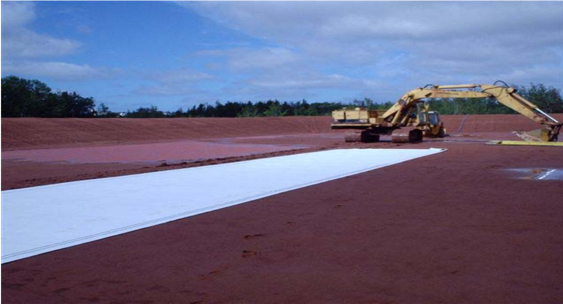
Photo courtesy of Scott Costain, Arrow Construction Moncton office.
