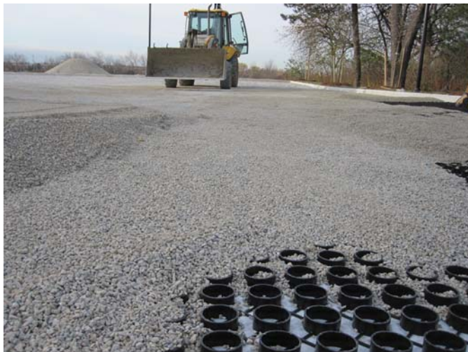
Gravel Paver – Fill cells with clean angular stone
