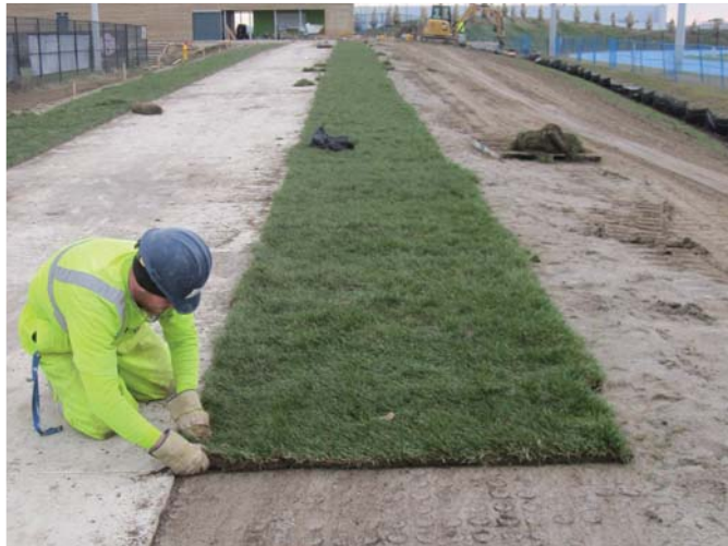
Grass Paver – Place sod over cells filled with clean concrete sand
