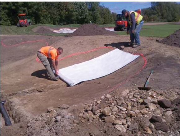
TerraBunker Panel – 5ft x 14ft – Weight 1 lb/sqft – no staples required.
