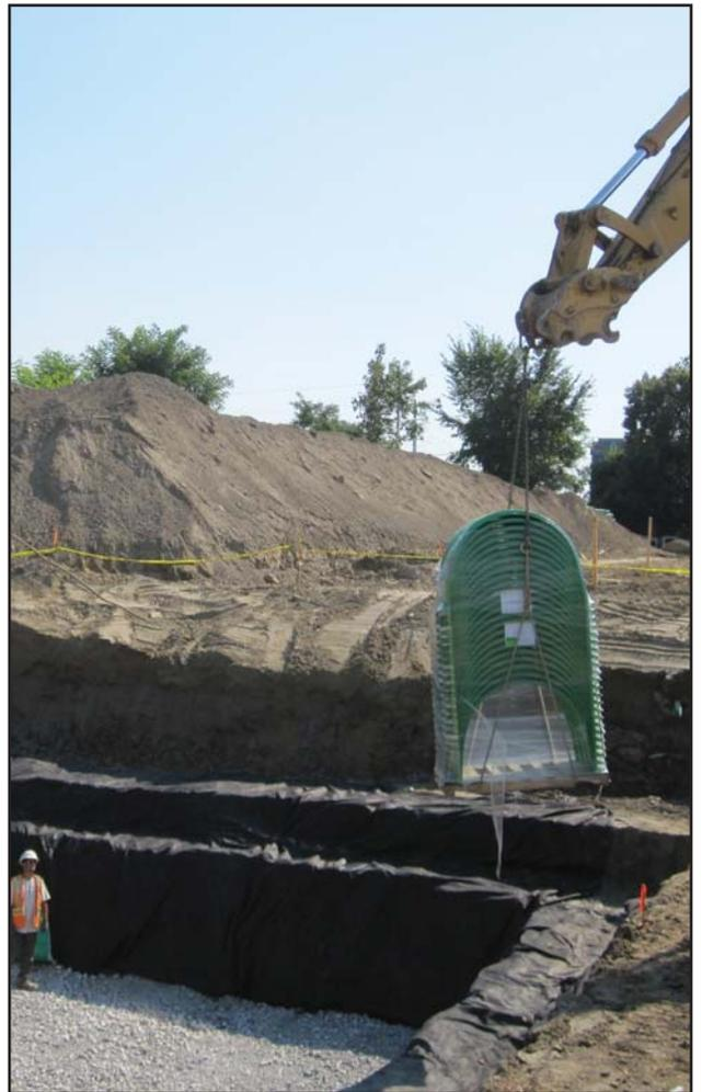
152mm of clear stone bedding. Carefully lowering skid of chambers in the trench
