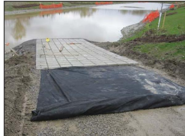
Filter fabric over compacted granular base
