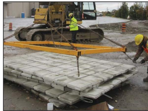
Attaching the lifting loops to the spreader bar
