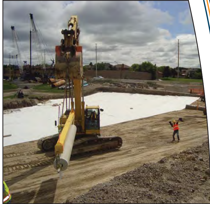
Bentofix deployment proceeding with ease.
