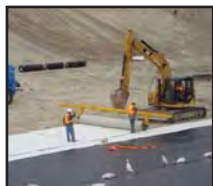
One foot cover soil being placed over the GCL.
