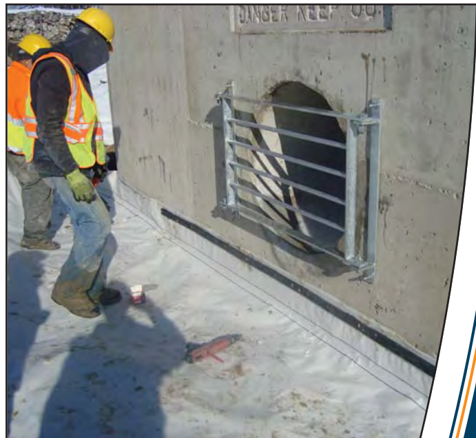
Nailed batten bar strips GCL-Concrete connection.
