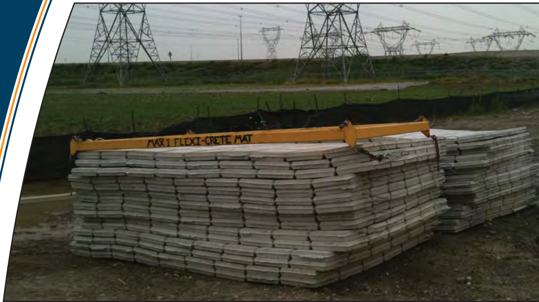
Panels of FLEXICRETE® on site
