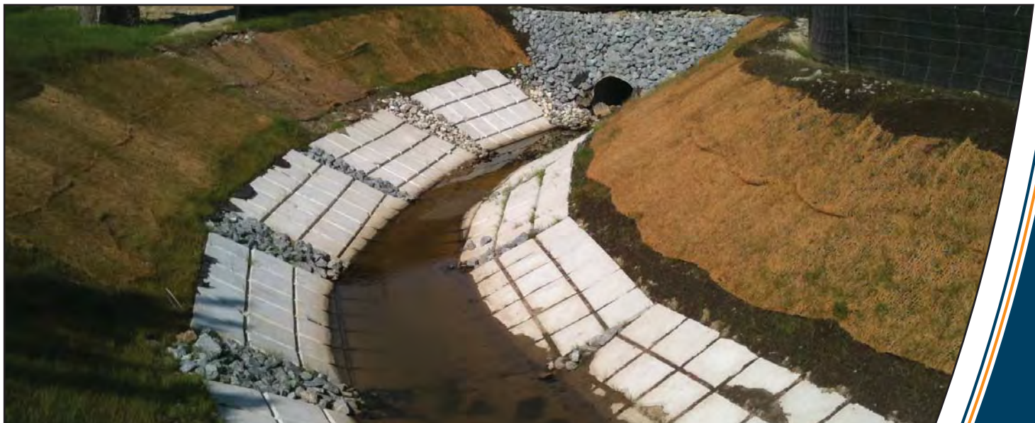
Outlet of culvert
