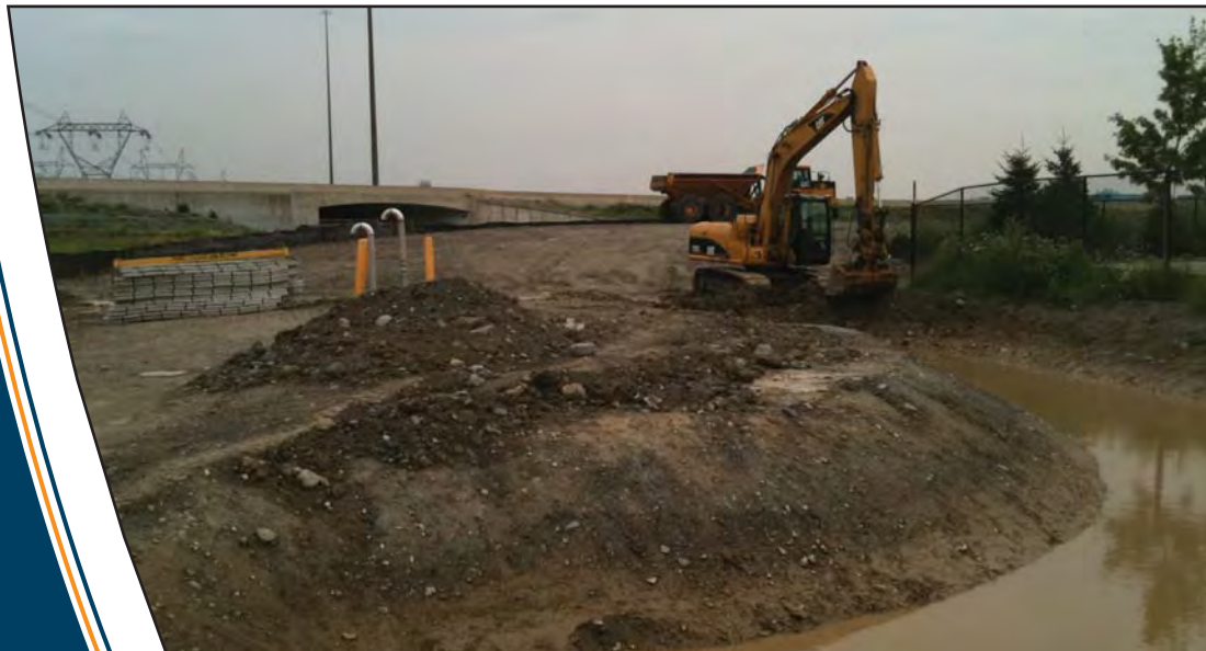
Excavation of channel
