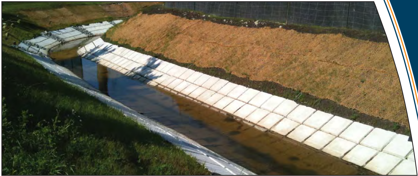
Erosion control blankets on the side slopes of the channel
