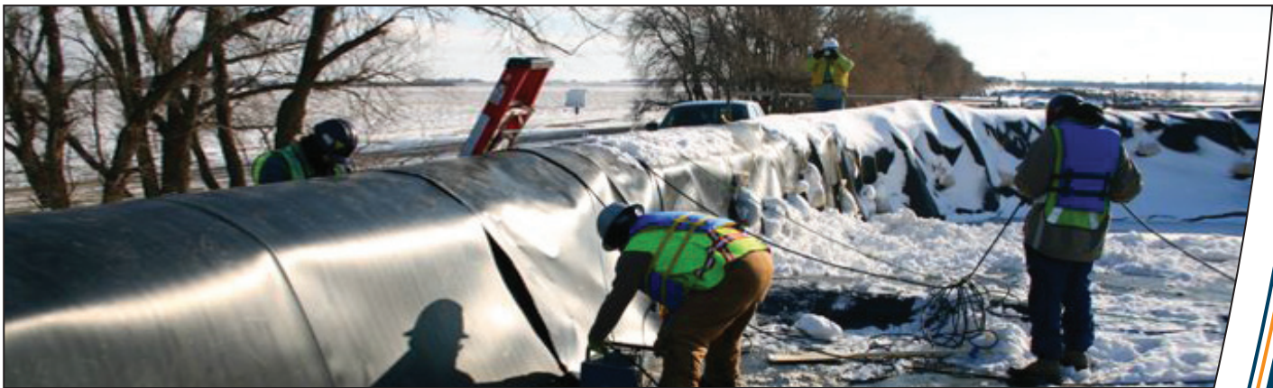
Terrafix crew completed the work despite the inclement weather
