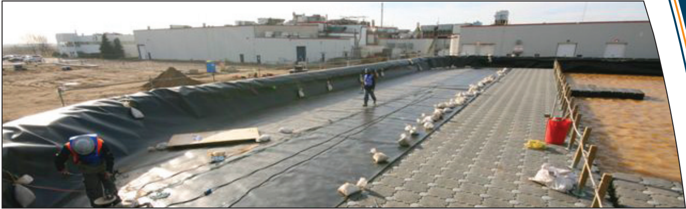
Floating platform used for installation
