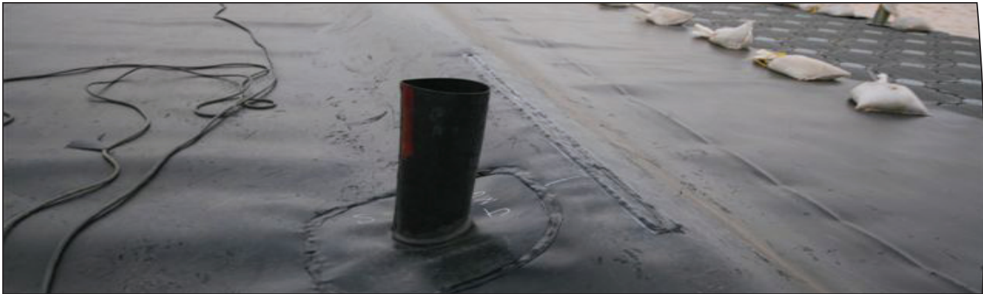
Vents were installed on the Floating Cover
