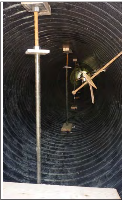
Jacks to anchor Weholite pipe to the bottom prior to grouting
