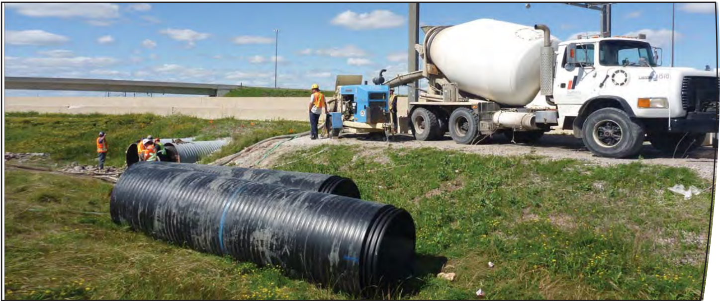
Grouting annular voids between Weholite pipe and existing CSP.
