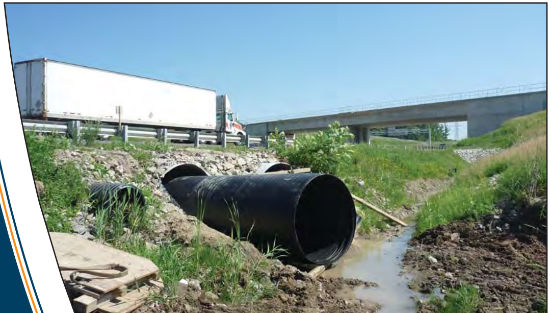
Sliplining 1372mm dia. Weholite pipes underneath Hwy407 at Appleby Line.
