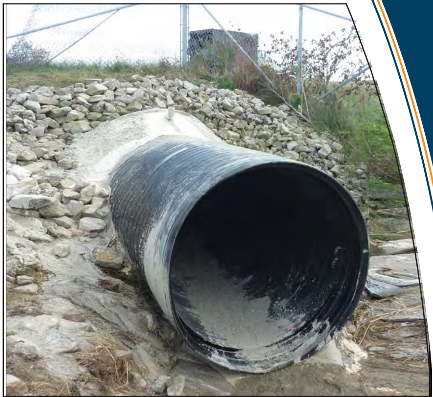
Bulkheads formed to contain the pumped grout.
