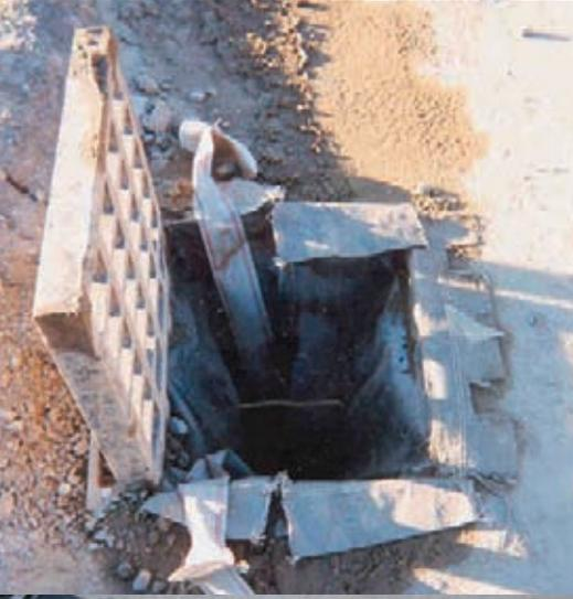
SILTSACK® is a sediment control device used to prevent silt and sediment from entering your drainage system. SILTSACK® traps the silt / sediment but allows water to pass through into the sewer. SILTSACK® can be used as a primary or secondary sediment control device to prevent failure of drainage system due to clogging with silt / sedimentation. Maintenance of the SILTSACK® on a regular basis will ensure that the SILTSACK® will function properly.
