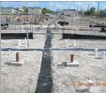
terrafix® provides the industry standard in gas vapor membrane technology, designed to eliminate vapor intrusion into structures built on brownfields or any other contaminated sites (i.e. former landfills, buried organics or fill and manufacturing facilities, former dry cleaners and gas station sites).
