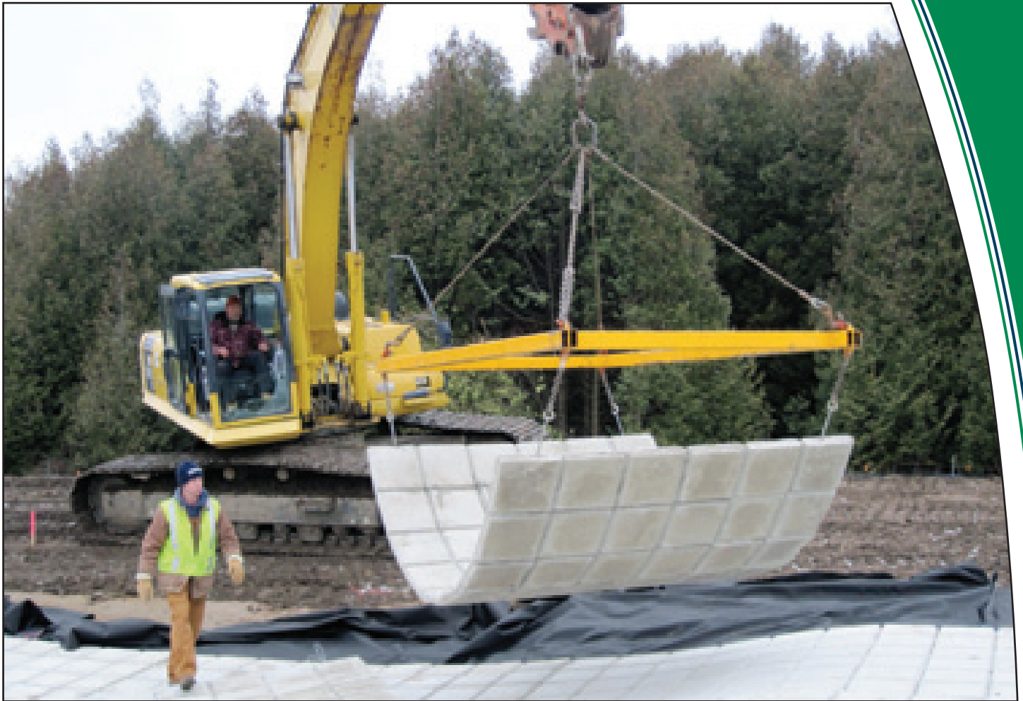
Lifting a panel with the spreader bar
