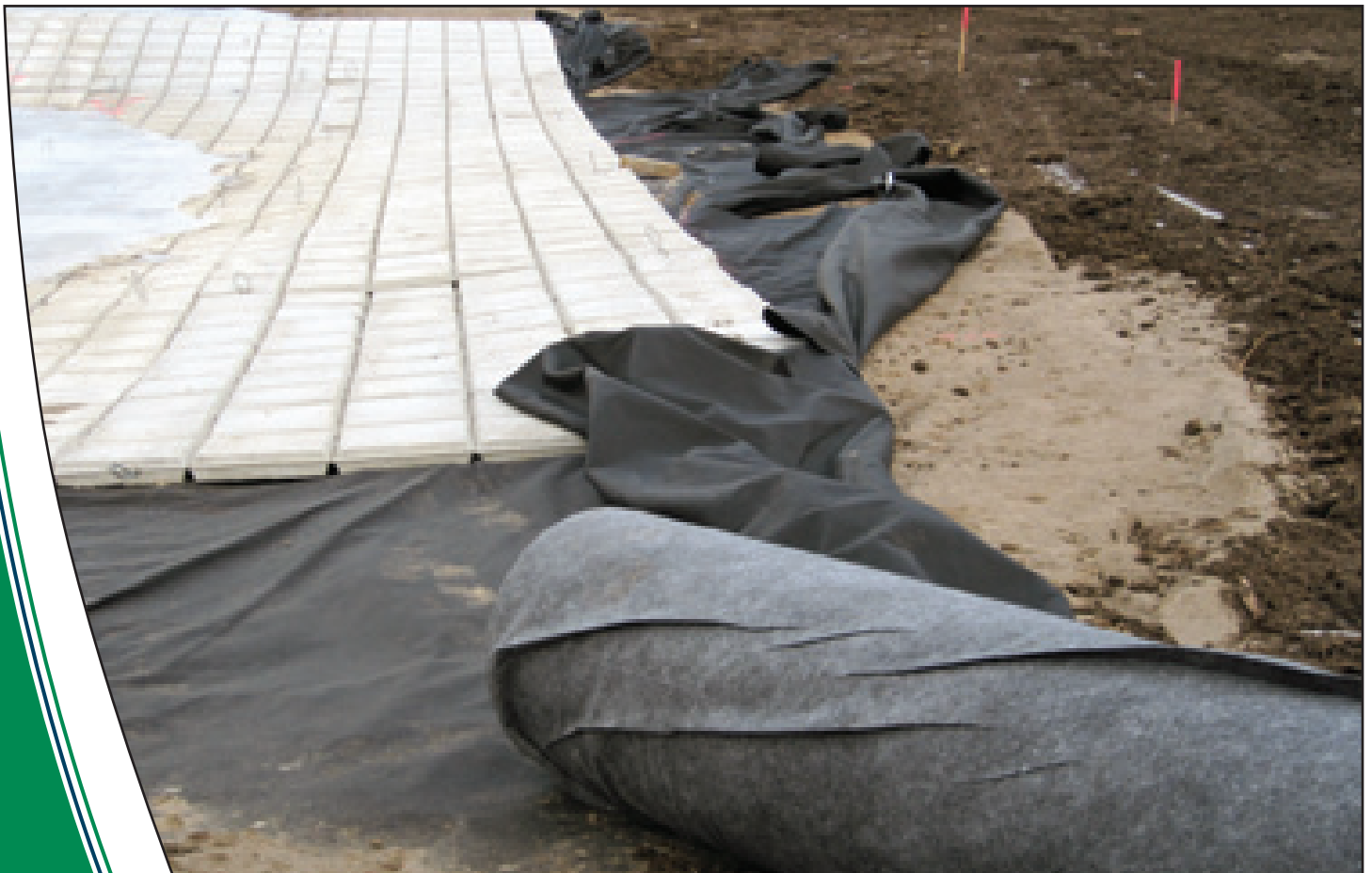
Non-woven geotextile laid over compacted base
