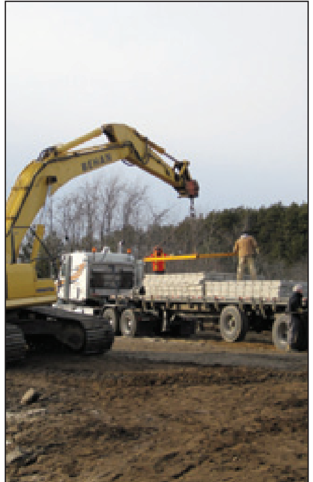
Lifting panels off of flat bed truck
