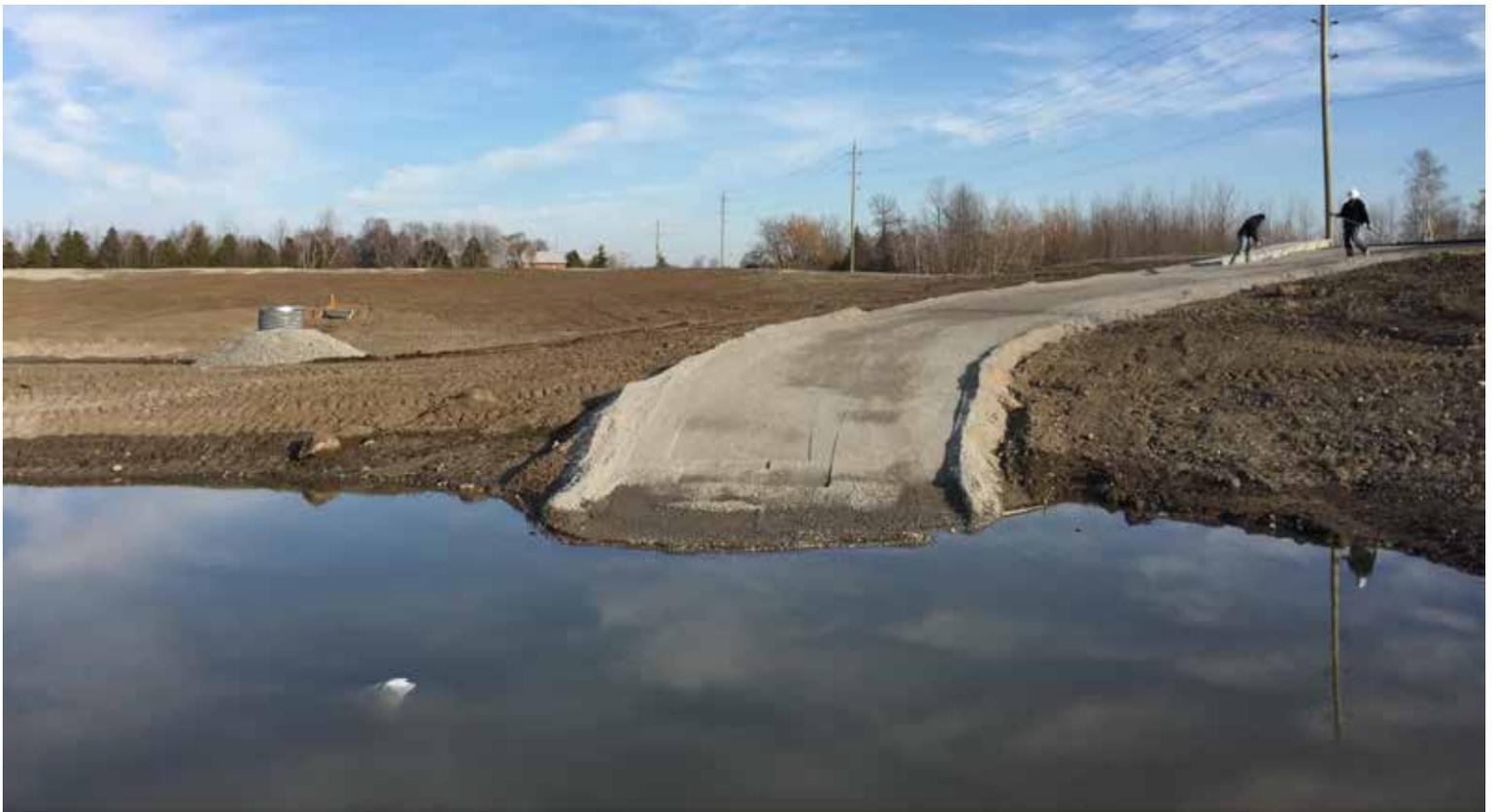
FLEXICRETE is a system of solid concrete blocks connected together to form continuous inter-connected areas. Concrete strength used is 30MPa or higher in accordance with Canadian Standards CSA-A23. Galvanized mesh reinforcement wires (8 gauge) are cast into the blocks. The standard block size is 400mm x 400mm x 81mm.
