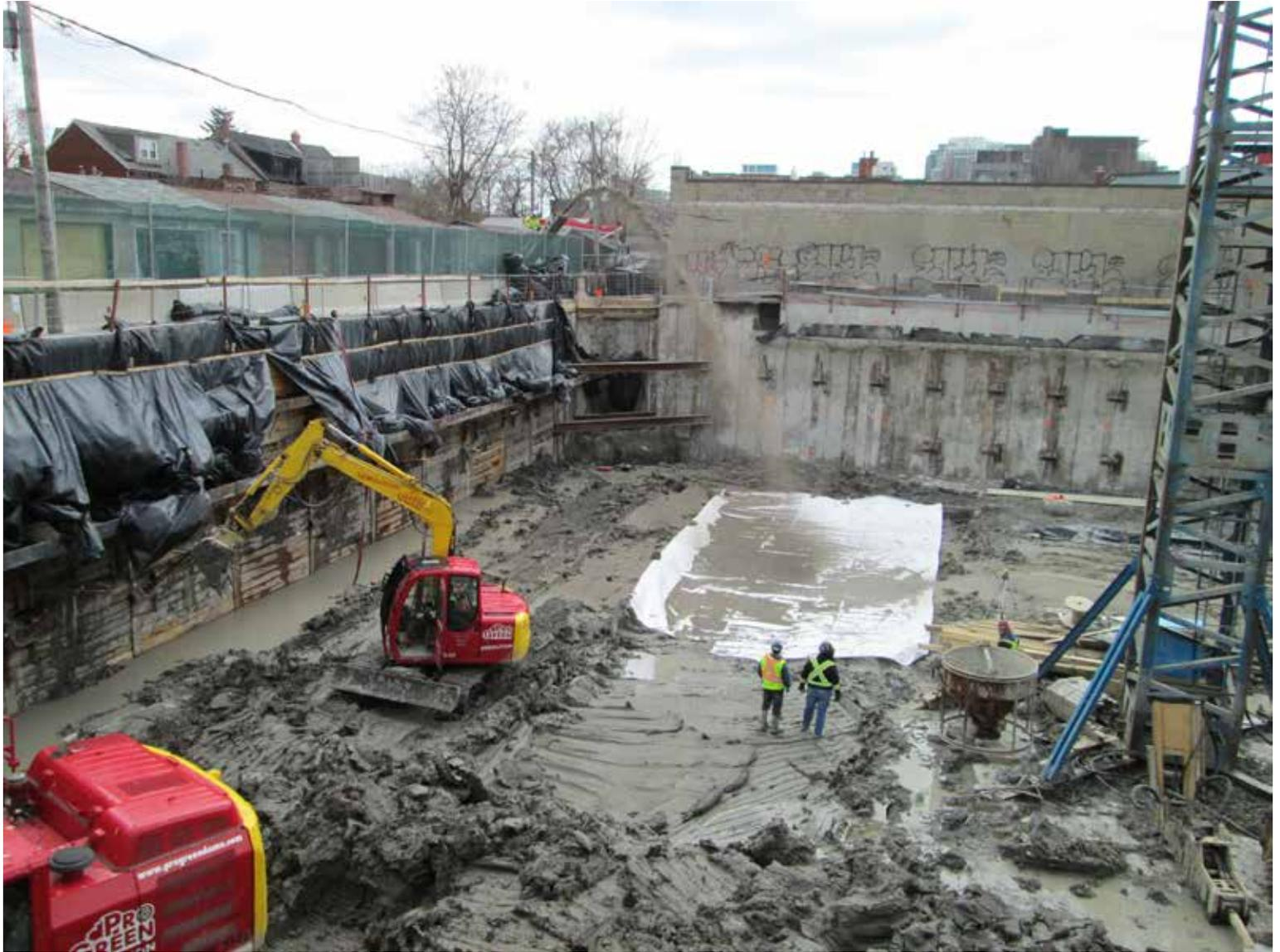
Saturated Clay Subgrade with very low bearing capacity
