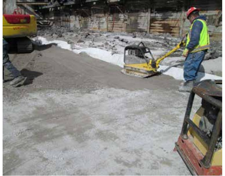
Aggregate flung and compacted to ensure interlock and compaction
