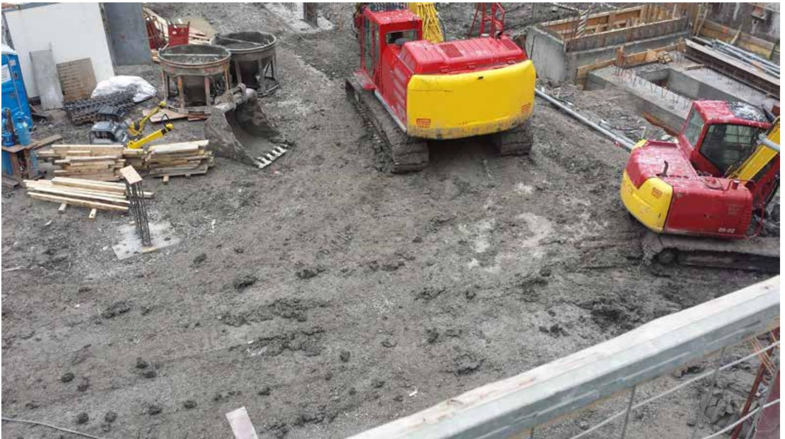
Completed work platform supporting heavy equipment at excavated depth
