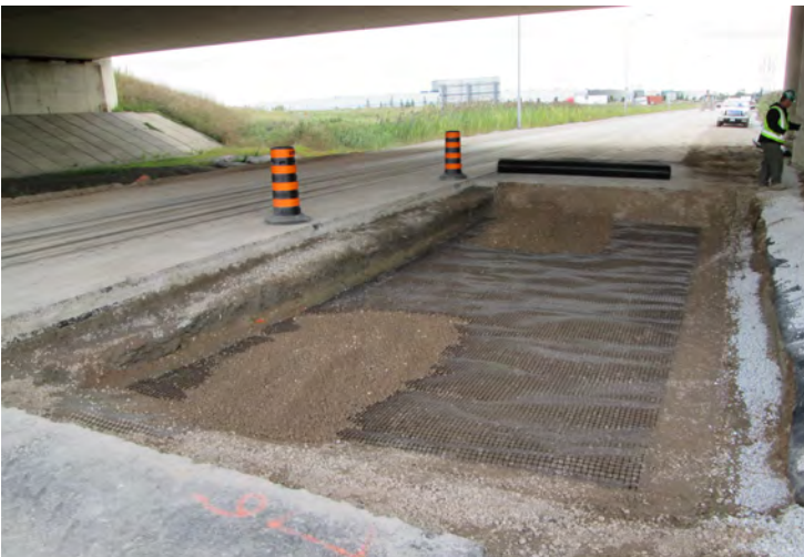
TBX2500 laid out over excavated grade
