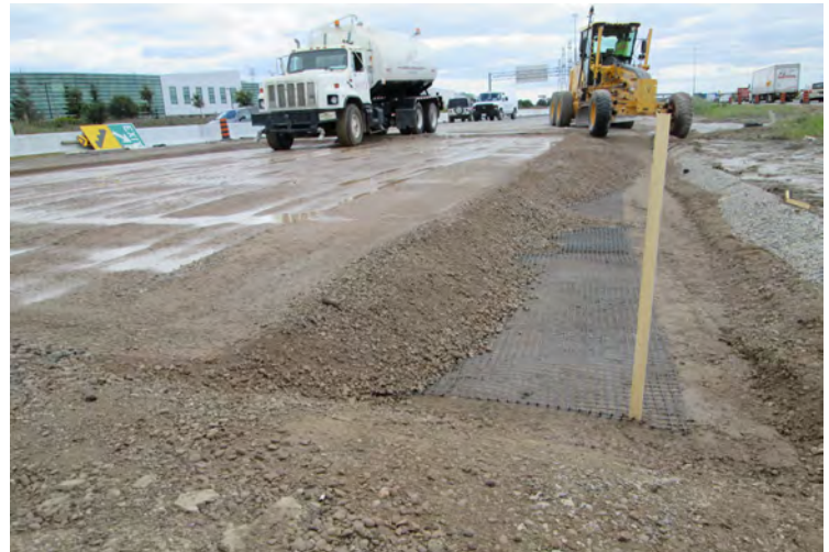
Structural fill laid and compacted on TBX2500
