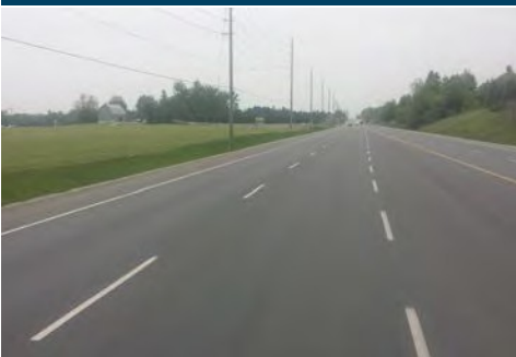
Completed Eastbound lane expansion
