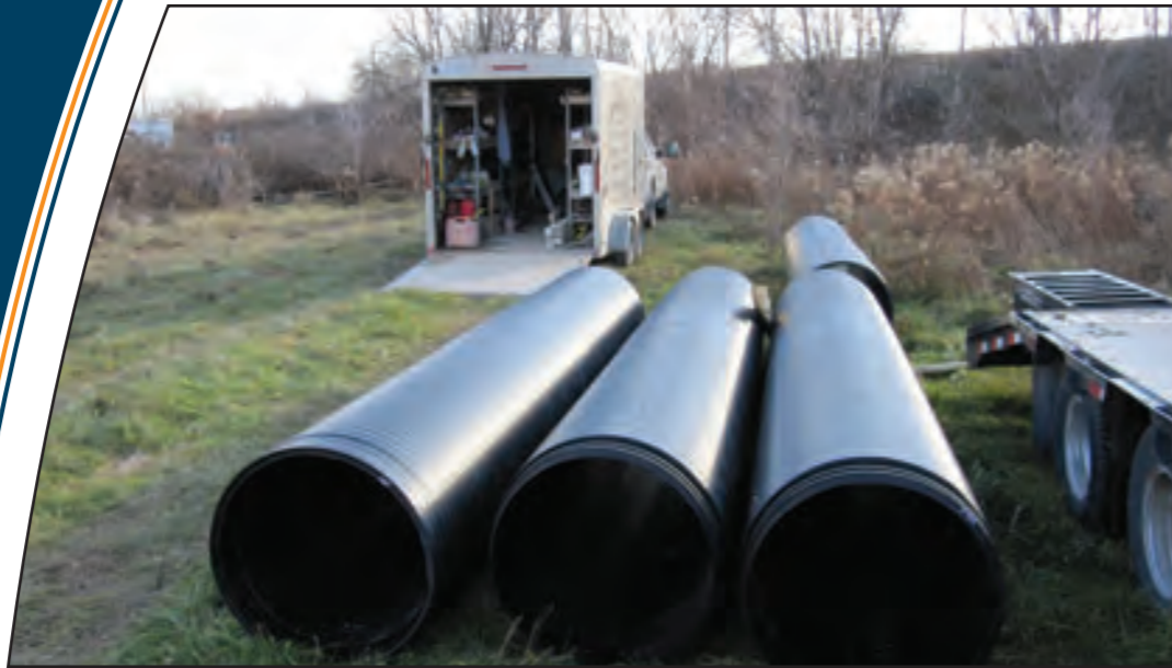
Delivered on site - 690mm dia Weholite, RSC160, 5.03m lengths, threaded ends.
