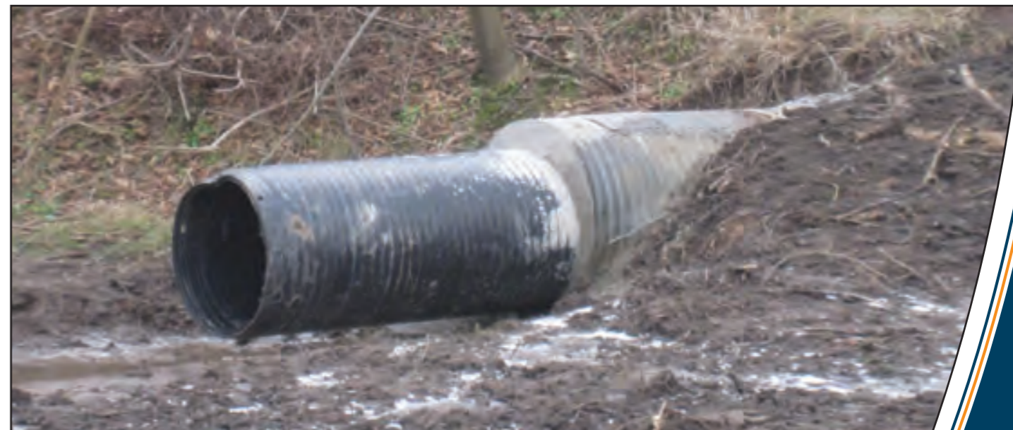
Concrete bulkhead to contain the grout within the annular voids.
