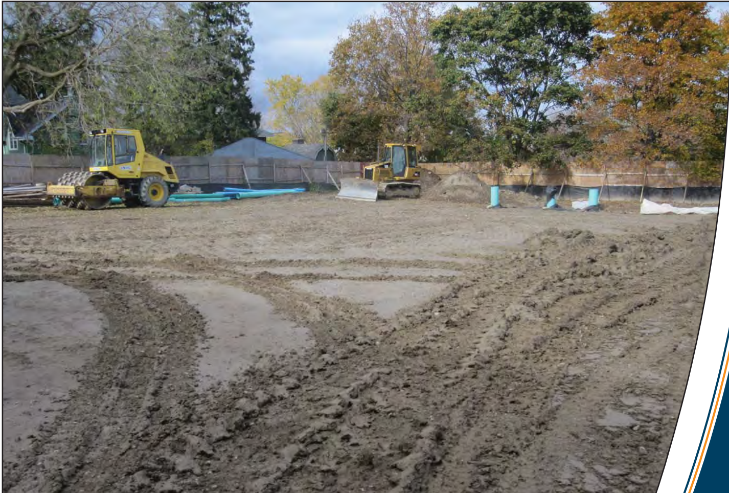
Compaction of backfill material
