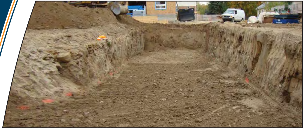
Excavation of trench
