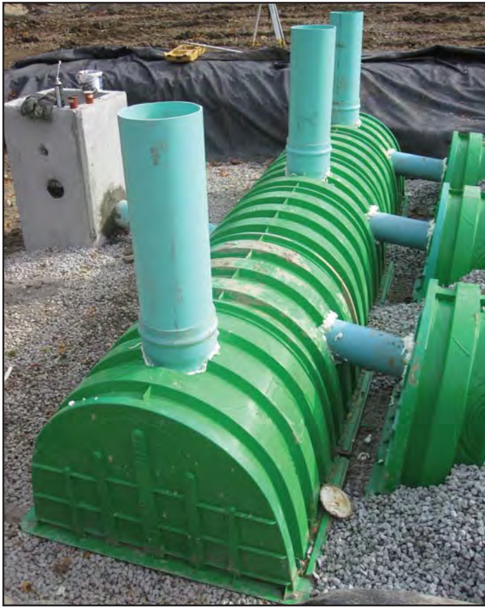
300mm inspection ports above the header row
