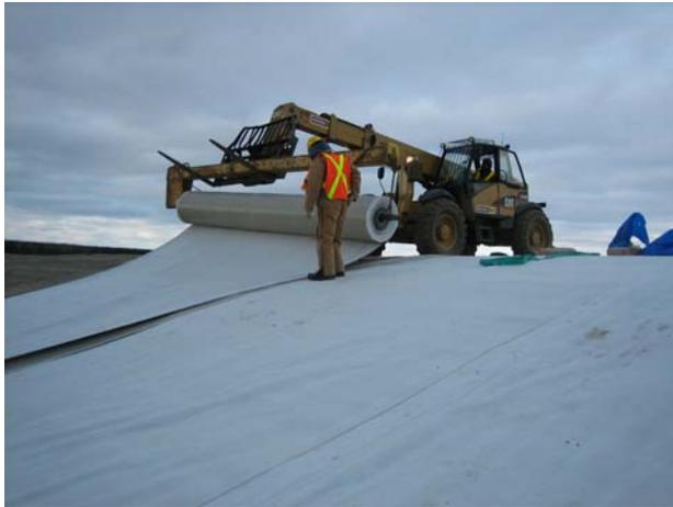
Figure 3. Deployment of the GCL. One foot overlap being done. Polypropylene side of the GCL facing down.
