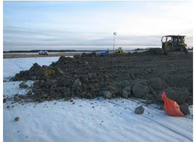
Figure 5. Clay being applied over the GCL.
