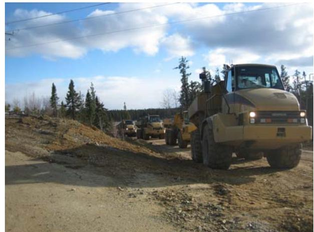
Figure 2. Hazco's truck fleet carrying the clay from a nearby clay source available on site being transported as a cover soil over the geosynthetic clay liner.
