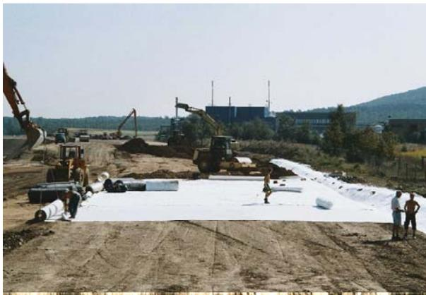
Figure 5. Installation of geosynthetics in the infrastructure sealing application by-pass road B 82n Langelsheim, Germany
