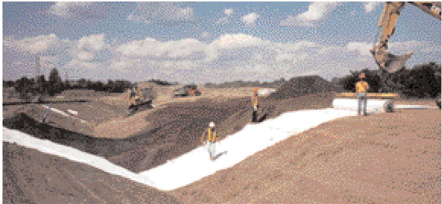
**Photo 1.** Installation of the geosynthetic clay liner over the existing landfill, 2001. View of the stormwater channel.
