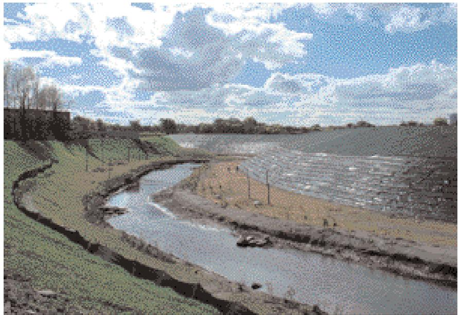
**Photo 4.** New creek and stabilized slope with vegetation growth in progress. The geogrid system had a built-in erosion blanket that was also hydroseeded.
