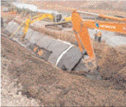
**Photo 2.** Installation of the pipe collection system along with the lining system, which included the use of a 60 mil HDPE, GCL, and drainage net.
