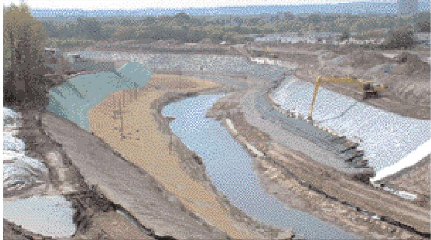
**Photo 3.** Construction of the slope along the landfill included the use of drainage net to collect the contaminants, a GCL, and a geogrid wrap system to ensure slope stabilization.
