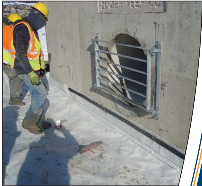
Nailed batten bar strips GCL-Concrete connection.
