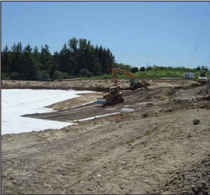
One foot cover soil being placed over the GCL.
