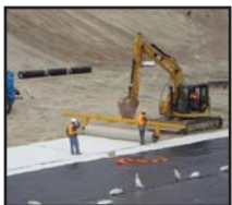
One foot cover soil being placed over the GCL.
