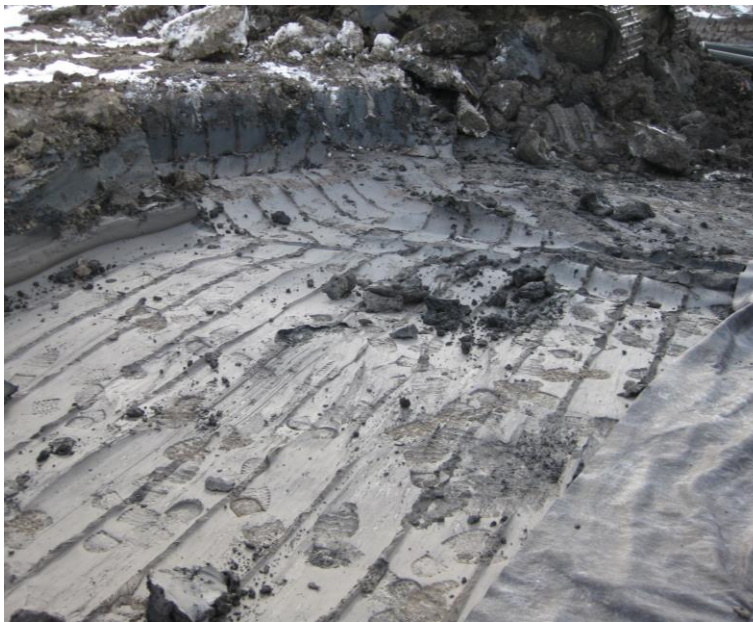
Construction Site – Sobeys'- St. Catherines
