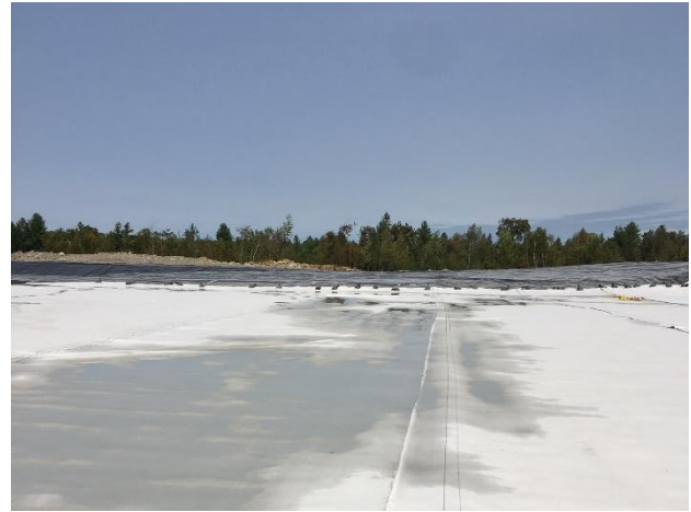
Figure 4. Premature Hydrated GCL on a landfill cell project from an afternoon thunderstorm/rainfall event.
